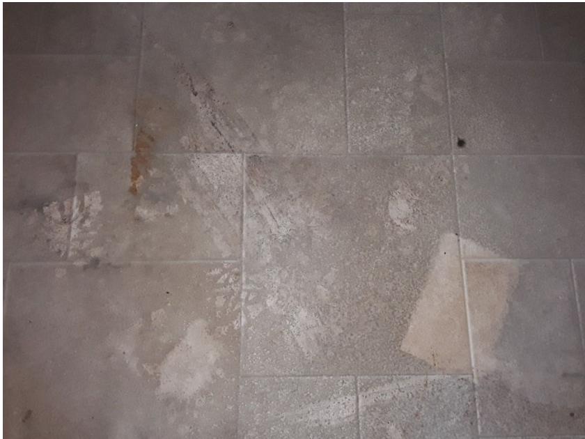
View of Tan Square Pattern Sheet Flooring and Adhesive (HA13)
