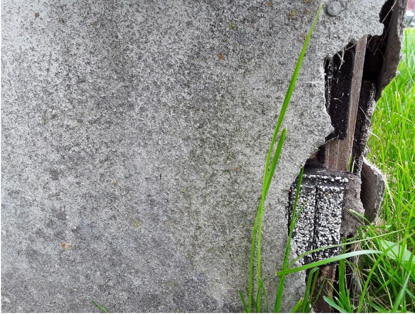
View of Asbestos Containing Exterior Transite Skirting (HA8)
