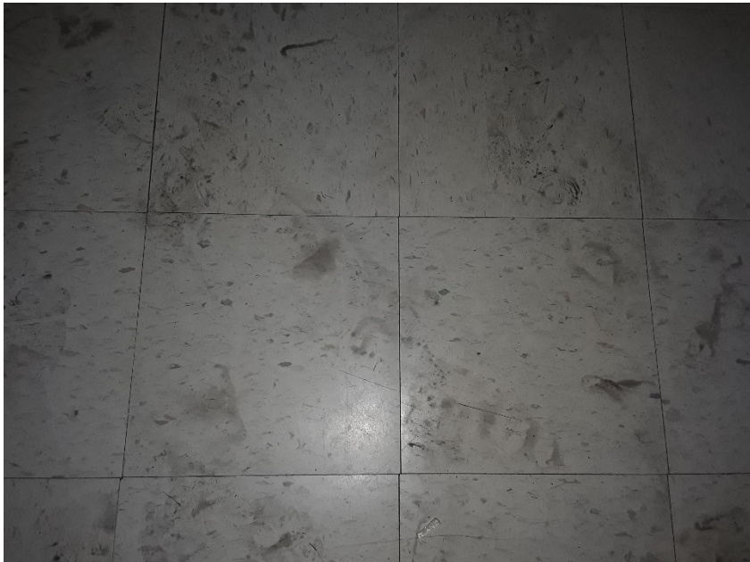
View of 12" x 12" White with Red and Blue Specks Floor Tile and Mastic (HA11)
