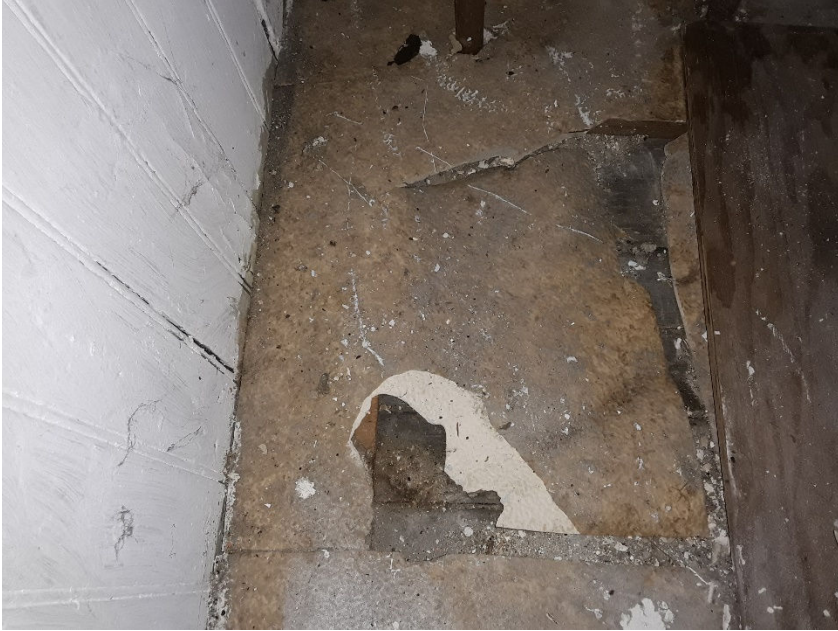
View of Yellow Flooring Under Wood Plank Flooring (HA6)
