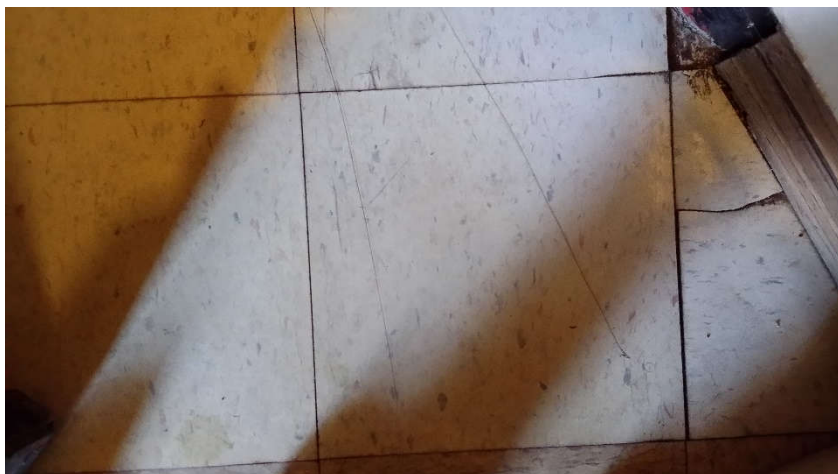
View of 12" x 12" White with Red and Blue Specks Floor Tile and Mastic (HA11)
