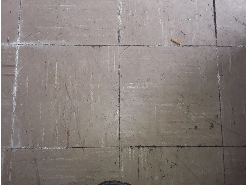
View of 12" x 12" Grey Mottled Floor Tile and Mastic (HA10)
