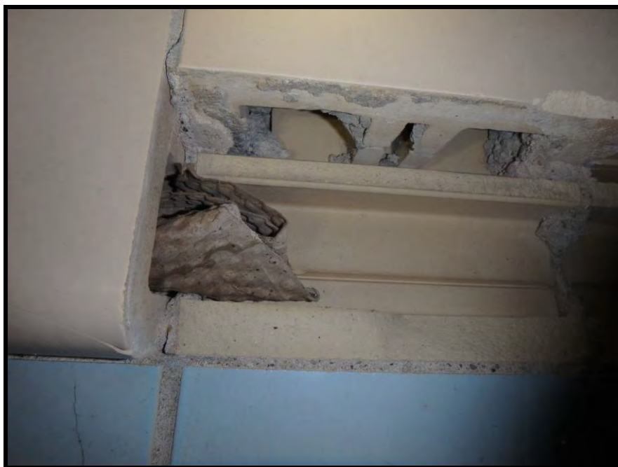
INTERIOR VIEW OF POOL AREA BROWN PAPER WITHIN GLAZED WALLING (HA-88)
