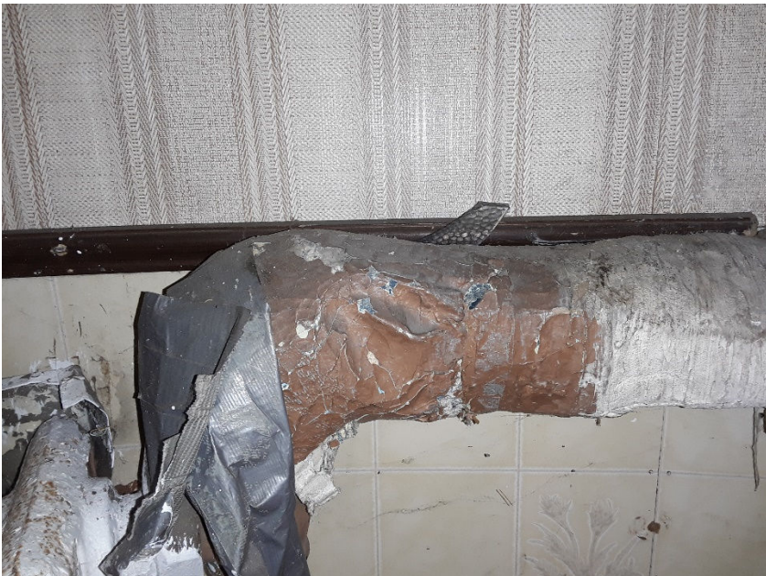
View of Asbestos Containing Mudded Fittings Associated with Straight Pipe Insulation (HA1)
