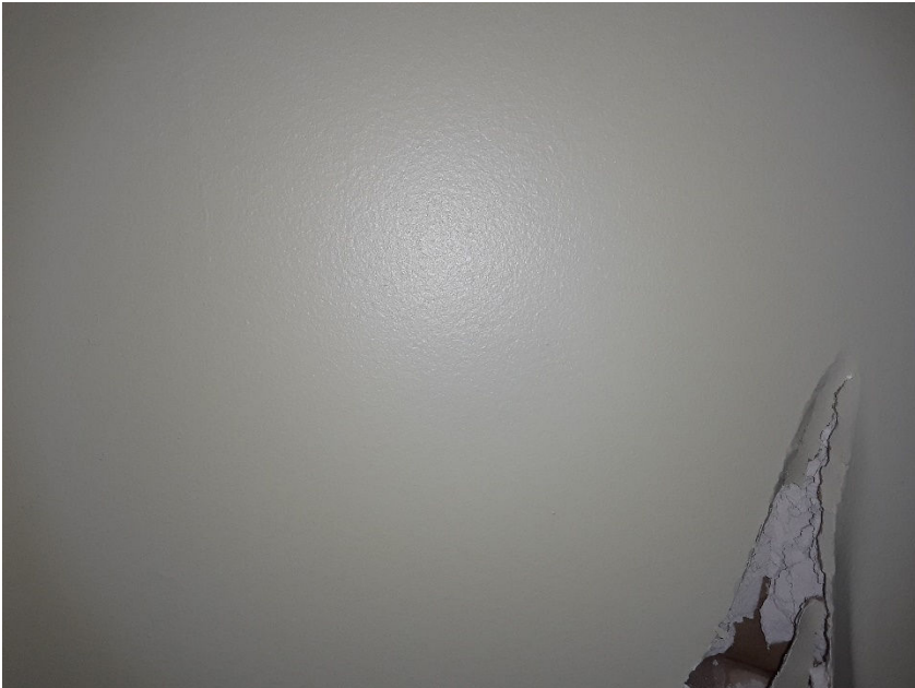
Typical View of Light Green Interior Paint on Drywall (PC-3)
