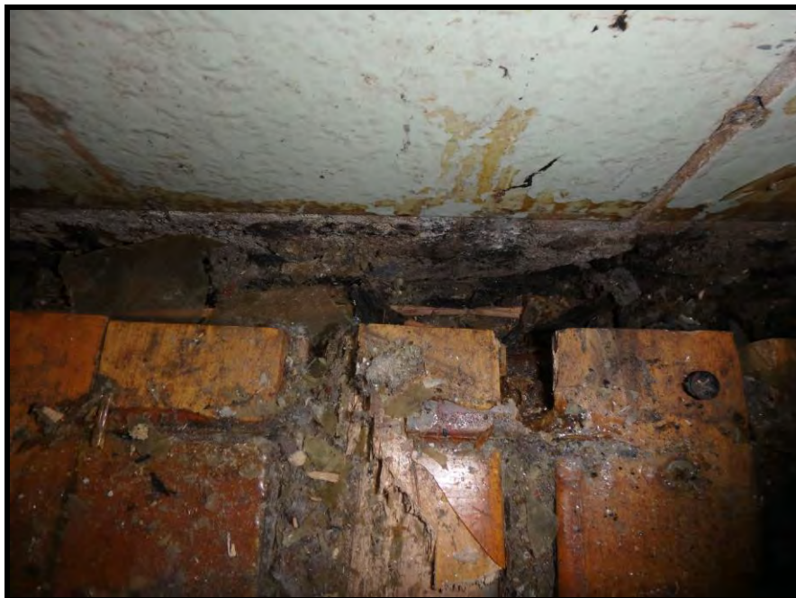
INTERIOR VIEW OF GYMNASIUM FLOOR BARRIER PAPER (HA-62)
