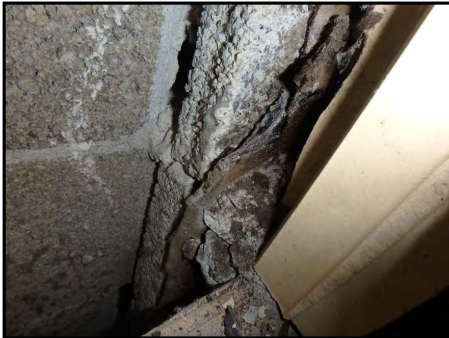
INTERIOR VIEW OF POOL AREA BLACK PAPER WITHIN PERIMETER WALL (HA-87)
