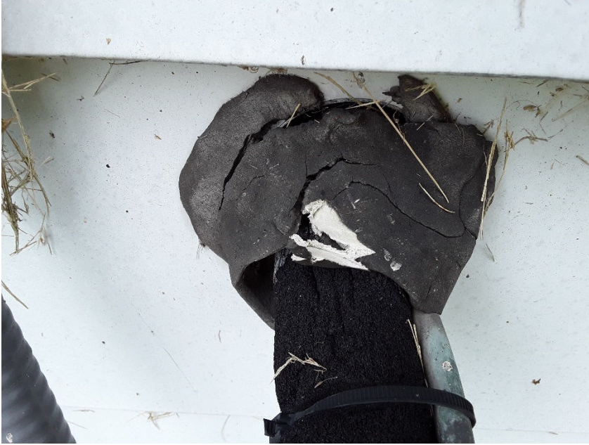
View of Light Grey Exterior Pipe Penetration Caulk (HA16)
