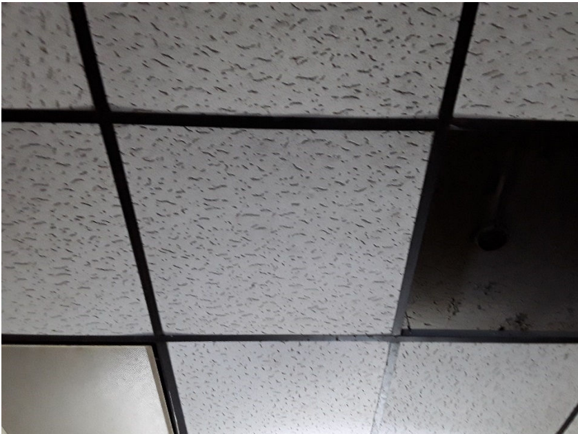
View of 2' x 2' Ceiling Tile with Pinholes and Log Gouges (HA13)
