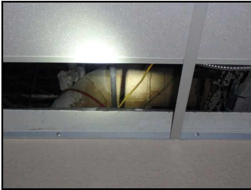
INTERIOR VIEW OF 1 ST FLOOR ABOVE CEILING SUSPECT TRANSITE PIPE (HA-84)
