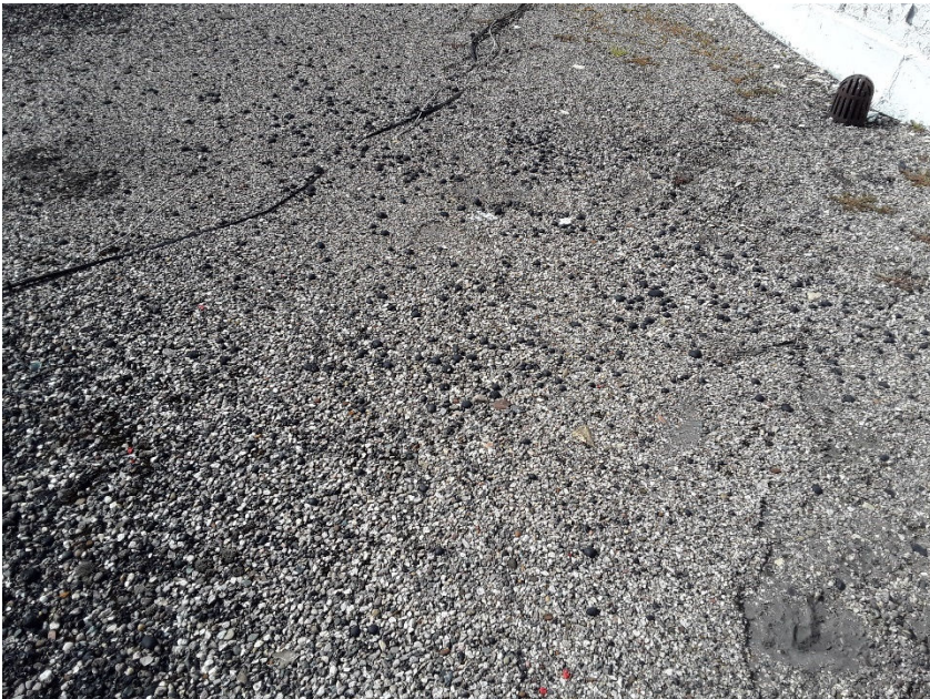
View of Asbestos Containing Flat Roofing Materials (HA15)
