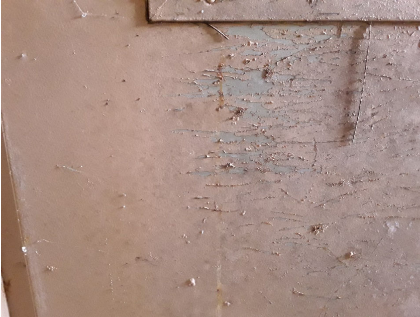
Typical View of Brown Interior Paint on Metal (PC-12)
