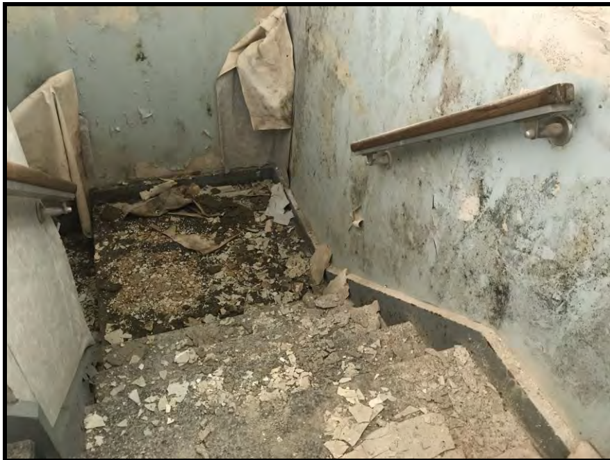
INTERIOR VIEW OF STAIRWAY AND MOISTURE INTRUSION
