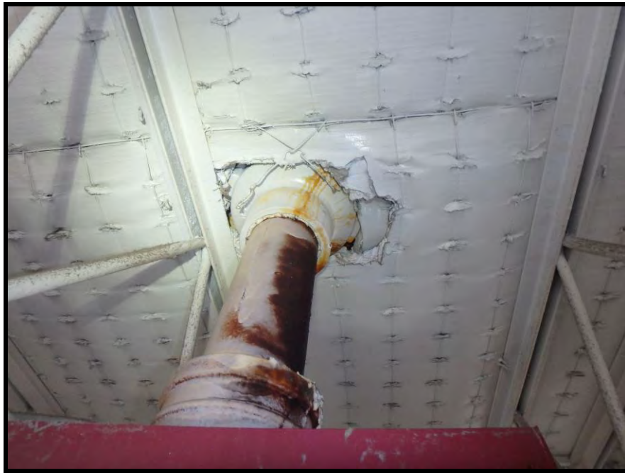
REPRESENTATIVE VIEW OF CEILING DRAIN MATERIAL (HA-70) AND PAPER TYPE CEILING MATERIAL (HA-71)
