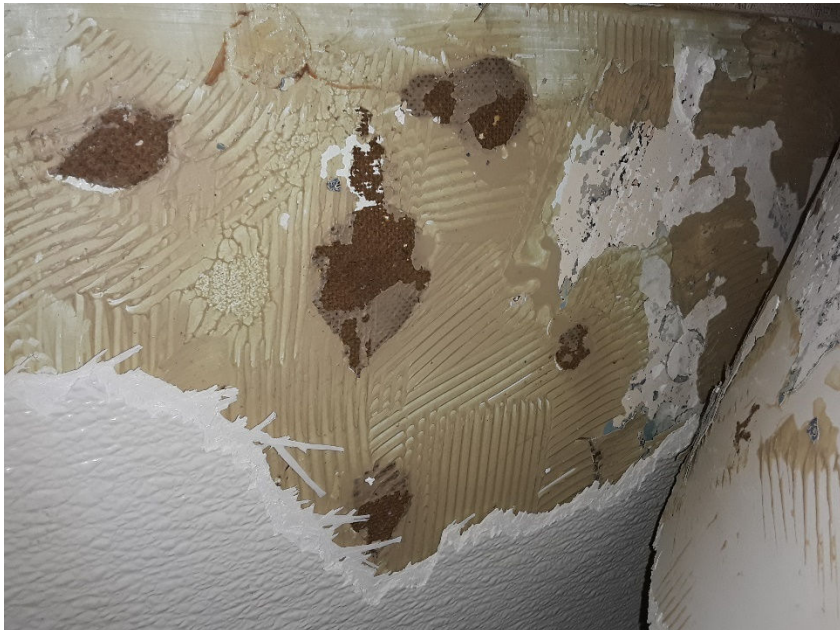
View of Fiberglass Reinforced Wall Panel Adhesive (HA23)
