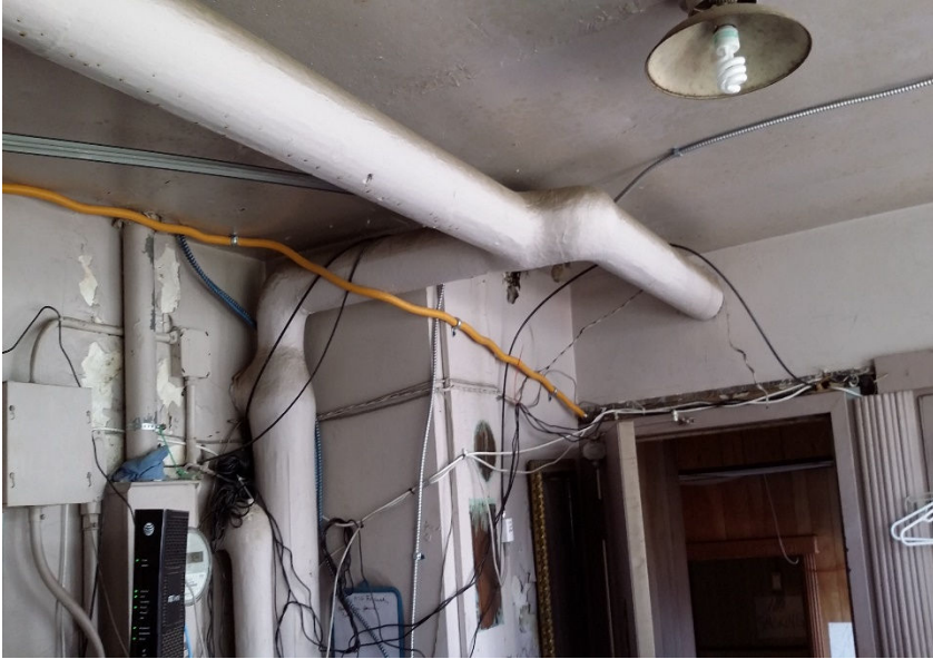
View of Asbestos Containing Straight Pipe Insulation (HA2)
