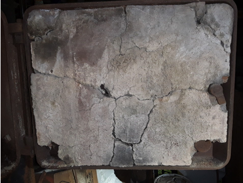
View of Asbestos Containing Boiler Door Insulation (HA4)
