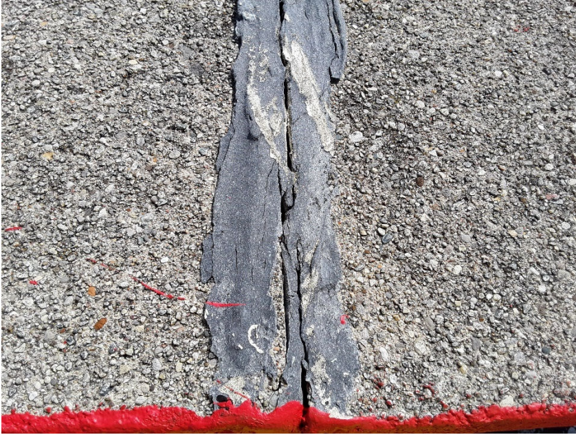
View of Asbestos Containing Black Exterior Building Caulk (HA26)
