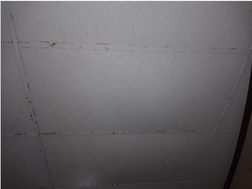
View of 2' x 4' Suspended Ceiling Tile with Long Gouges and Pinholes (HA7)
