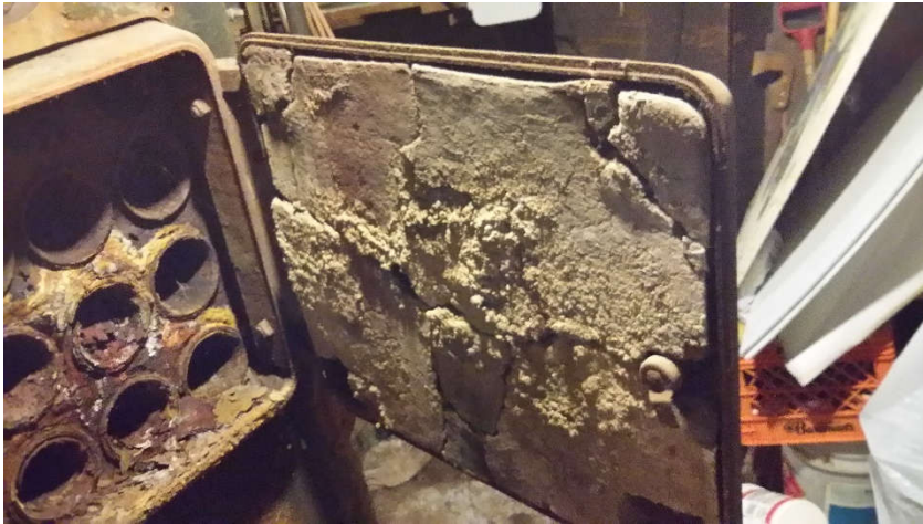
View of Asbestos Containing Boiler Door Insulation (HA4)
