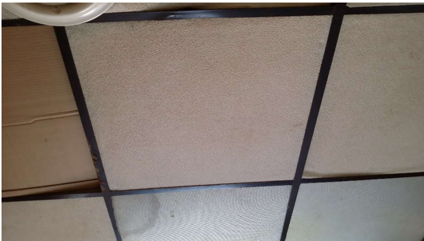
View of 2' x 2' Ceiling Tile with Pinholes and Long Gouges (HA13)
