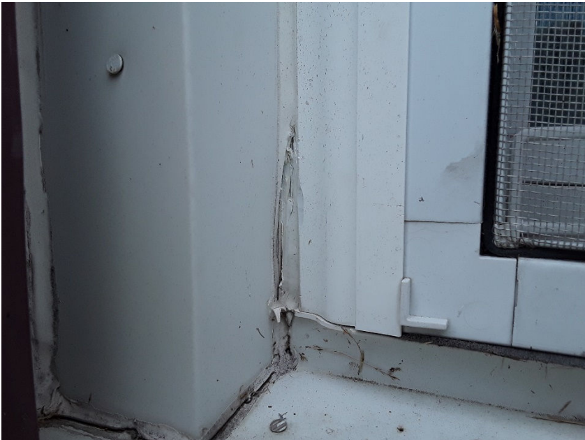
View of White Caulk Around Exterior Windows (HA9)
