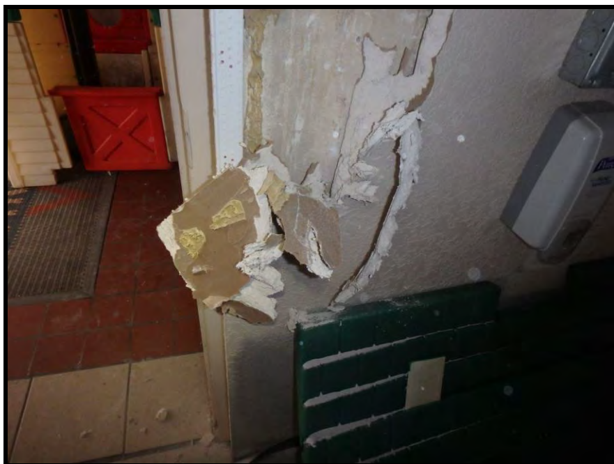
INTERIOR VIEW DRYWALL ADHESIVE (HA-50)
