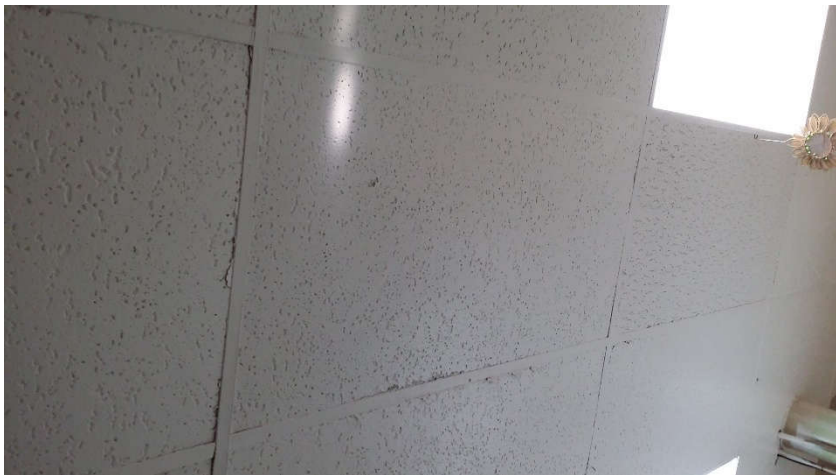
View of 2' x 4' Suspended Ceiling Tile – Long Gouges and Pinholes (HA7)
