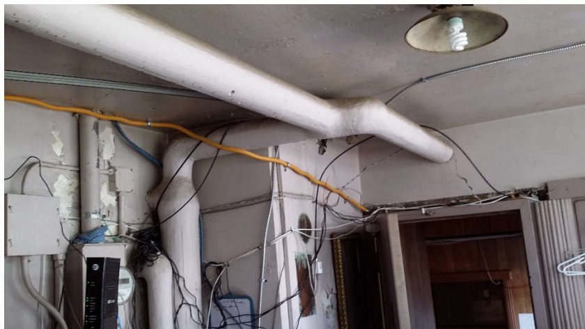
View of Asbestos Containing Straight Pipe Insulation (HA2)
