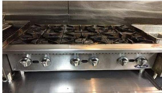
Equipment Elevated 4" Above Counter
