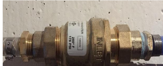
ASSE 1012: Used in place of ASSE 1022 devices except for carbonated beverage machines
